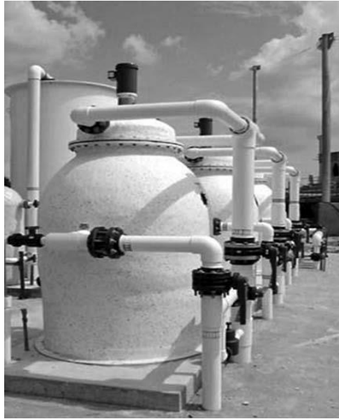
Figure 6. Propeller washed bead filter for biofiltration and solids capture (from Ebeling and Timmons, 2012).
