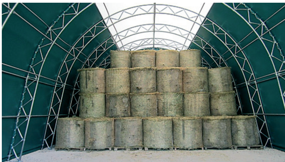
Slika 15. Skladišni objekt za biomasu (Izvor: https://torocorp.co.uk/Information/Articles/Biomass-BulkStorage-WhitePaper.html )
