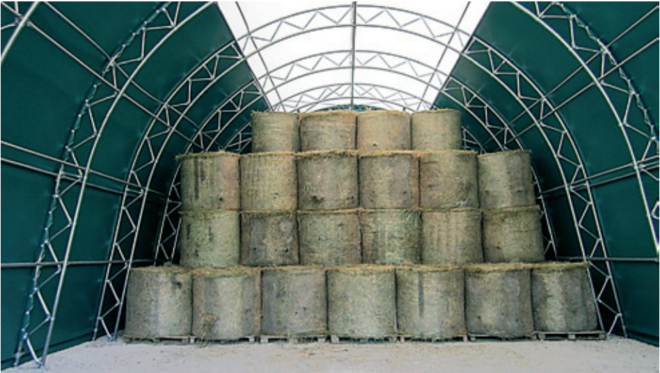
Slika 15. Skladišni objekt za biomasu (Izvor: https://torocorp.co.uk/Information/Articles/Biomass-BulkStorage-WhitePaper.html )
