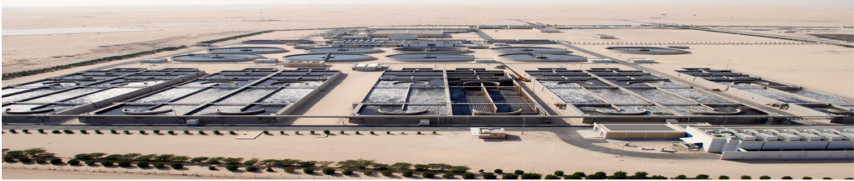
Figure 6. Sulaibiya wastewater treatment plant.
