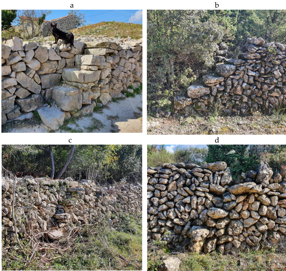
Figure 116. Forms of dry stone stairway access to agricultural parcels, in the environs of Stivan: a) and b) represent skalini ; c) and d) represent stalbice/stelbice (2020).
