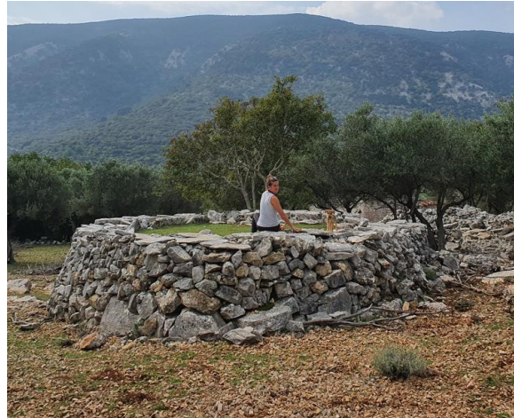
Figure 125. An elevated threshing floor in Veli Tržić: a) a rim covered in stone slabs, with a staircase, b) in the foothills of Osorščica (in the back) (2020)
