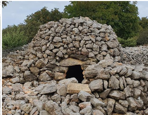
Figure 100. In its constructive form, this hut (located in the middle of the town of Cres olive grove) is similar to lime kilns; however, the entrance is too wide to make it one. It is unique in that its roof is made of stone slabs. (© Martina Krznarević, 2019)
