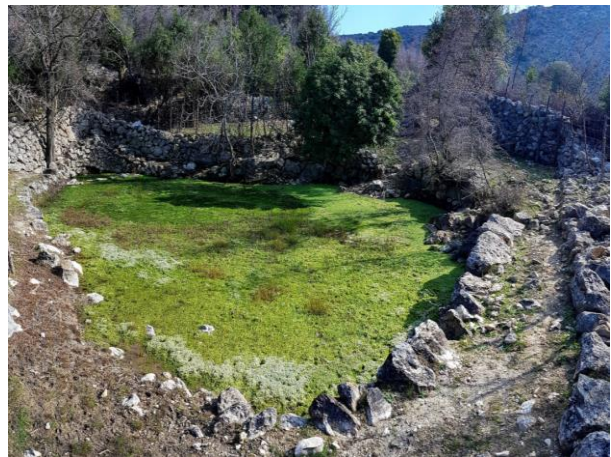
Figure 68. A community pond close to Vidovići, said to never evaporate fully, attached to an escarpment, lined with thick dry stone walls, and containing a paved stair entrance (2021)
