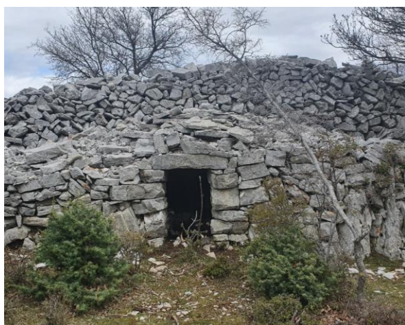
Figure 94. A dry stone hut, placed inside a clearance wall on the border of an isolated field among the pastures of Tramuntana (Ponehovice) (2021)
