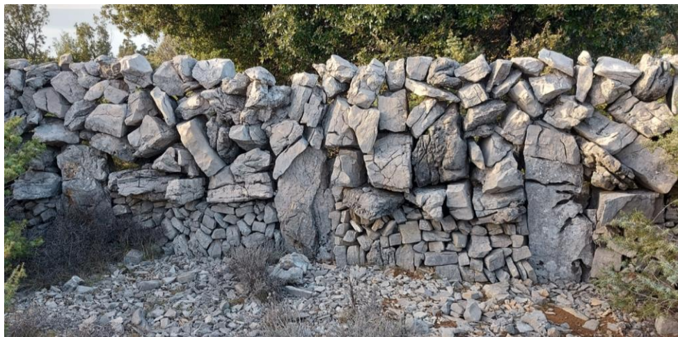
Figure 17. A dry stone wall built in a combined manner with stones ' na nož/na kultel ' in the Gerbin area (© Dorijan Lovrečić, 2021)
