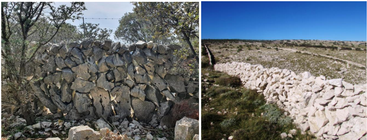
Figure 16. Single walls a) reinforced with wire (2021) and b) on the eastern shores of the island of Cres (2019)
