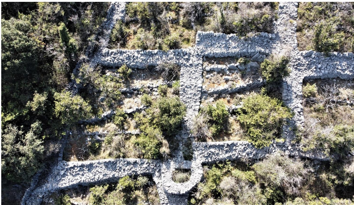
Figure 171. The Lovreški pattern consists of double dry stone walls which enclose a regular, rectangular area. The soil within is further stabilised by smaller dry stone structures (Pridanci), a line of transversely stacked stones. Remnants of a dry stone shelter (kućica) are seen at the bottom (2021).
