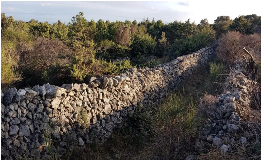
Figure 169. The area of Lovreški is heavily under vegetation, but the dry stone walls and the capstones are still in place (2020).
