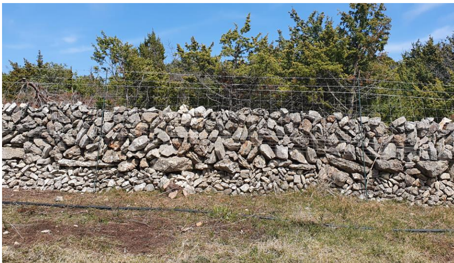
Figure 20. A combined dry stone wall reinforced by mesh to protect against allochthonous wild animals (Osor environs, 2021)
