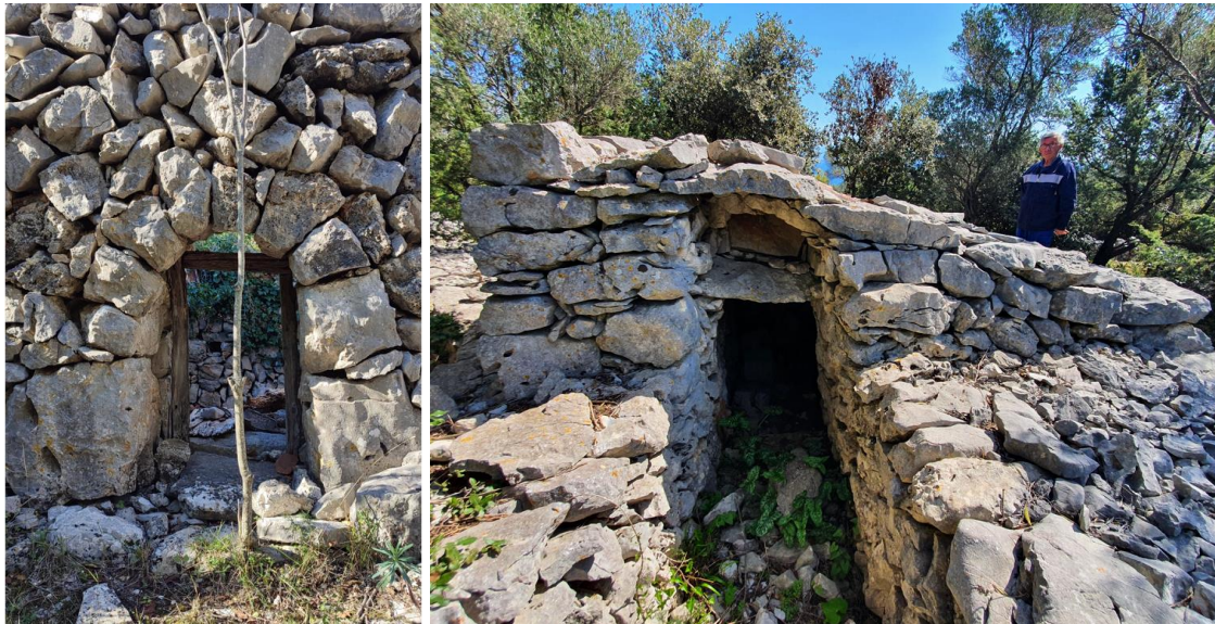
Figure 89. Dry stone livestock sheds and their dry stone constructive elements: a) an arch on the entranceway to a livestock shed, close to Lubenice (2021), and b) a livestock shed close to Arcić (Lovreški), with double lintel (2021)
