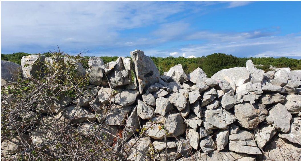
Figure 115. Different directions of the capstones above the dry stone wall separating the Ustrine and Belej commons mark the point up to which the shepherds of each common are responsible for its repairs (2020)
