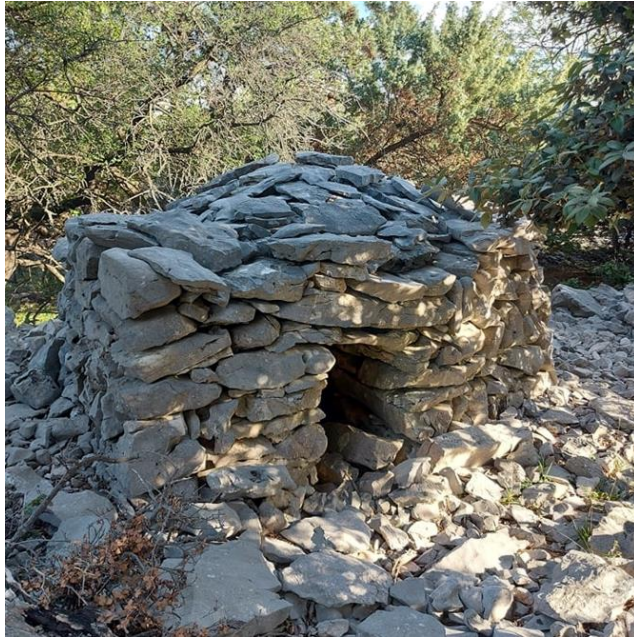
Figure 98. A dry stone hut with a square ground plan and a corbelled roof of stone plates, between the bays of Banja and Kruščica (© Dorijan Lovrečić, 2020)
