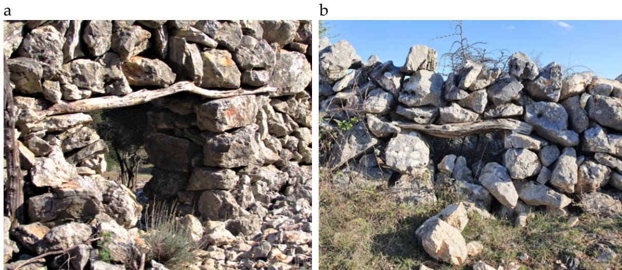
Figure 108. Lunky holes ( škùje ) covered with wooden lintels a) on the ‘Napoleon road’ north of the town of Cres (2017) and b) on the pathway to Zbišina (2021)
