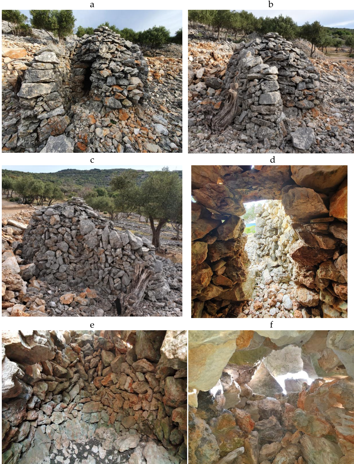
Figure 96. Different angles of the dry stone hut at the Stret locality, in the northern part of the Cres olive groves. Its interior is about 1.80 m high and allows for no more than one person to stand upright. It has one of the most preserved outer dry stone protective walls (2020).
