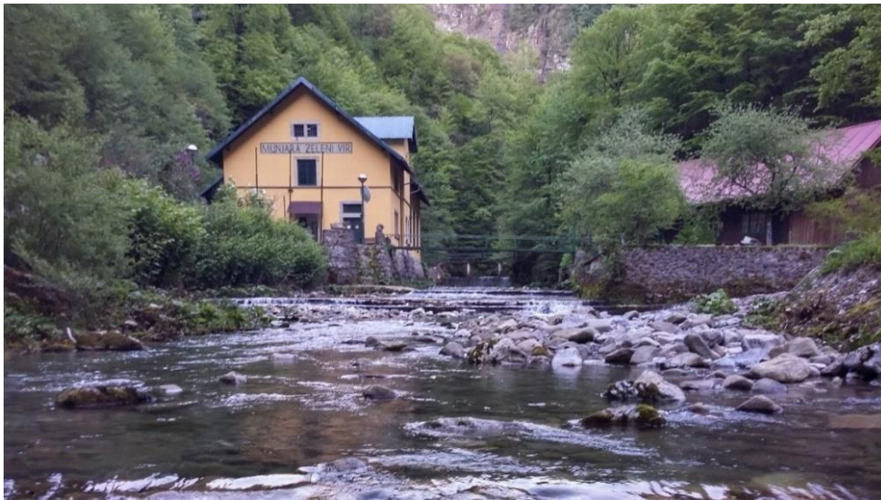
Figure 4. The Curak River and small hydroelectric power plant “Zeleni vir”.
