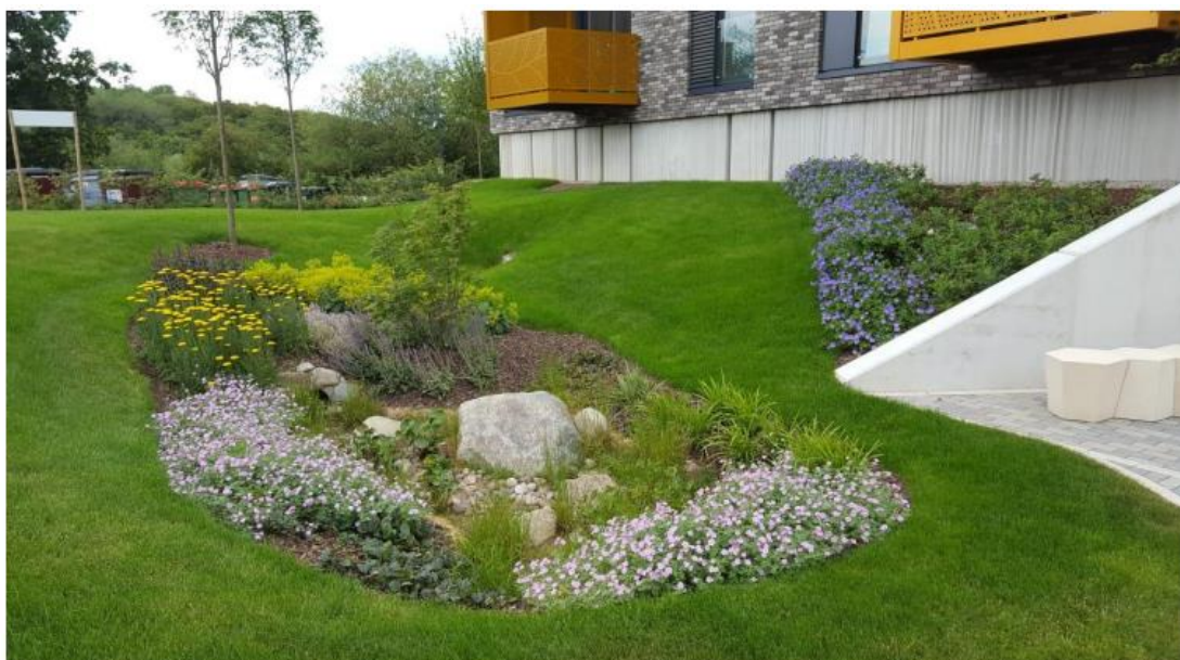
Slika 4.5.4. Prikaz kišnog vrta. Jehovah's Witnesses Britain Headquarters. Izvor: 001_29_04_20_jehovahs_witnesses_cheltenham_2020_awards.pdf - pristup 27.6.2022.
