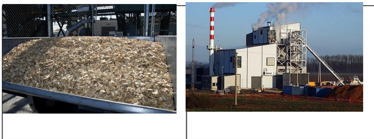
Figure 3.5.1. Cogeneration biomass plant facility Viridas Biomass, Babina Greda, Croatia ( https://bioenergyinternational.com/heat-power/27145 ;
