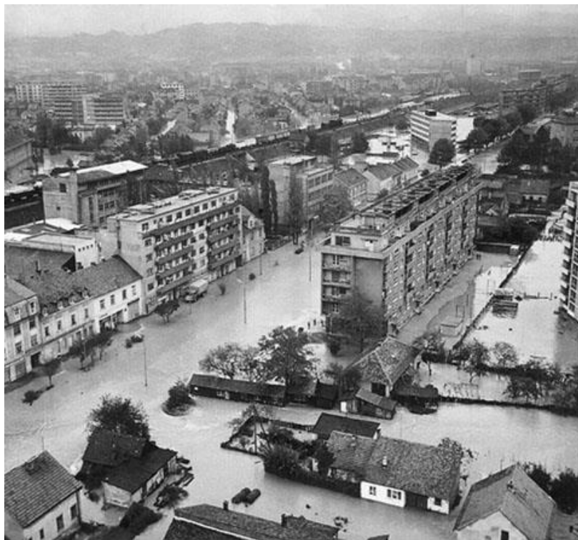
Figure 6. Flood in Zagreb in 1964
