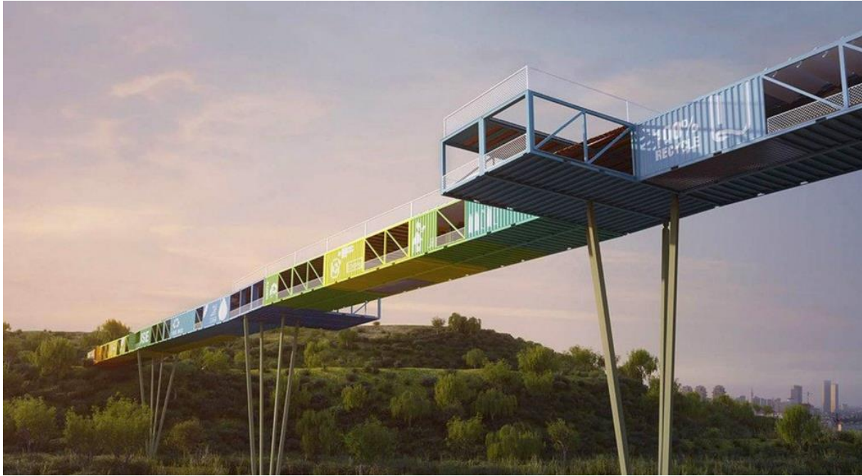
Slika 37: Most od kontejnera ( https://inhabitat.com/econtainer-recycled-shipping-container-bridge-to-provide-gateway-to-tel-aviv-arial-sharon-national-park/ )
