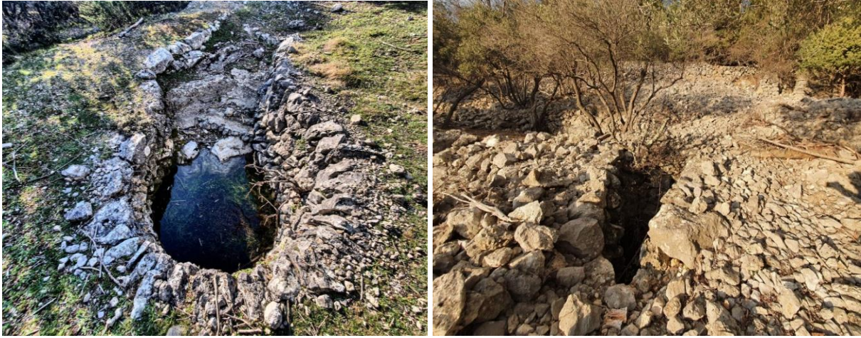
Figure 72. A dry stone pond in the locality of Sergovi. Access is enabled by stone stairs which were later partially concreted (2020)
