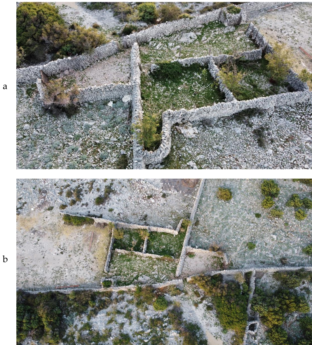
Figure 52. The multicellular sheepfold Mihojski . a) The two upper partitions are currently the only ones in active use. b) The pregrajčić is the wider space at the entrance to the mrgar , visible on the left side of the photograph. Two przgari are visible; the left one belongs to the Mihojski sheepfold (2020).
