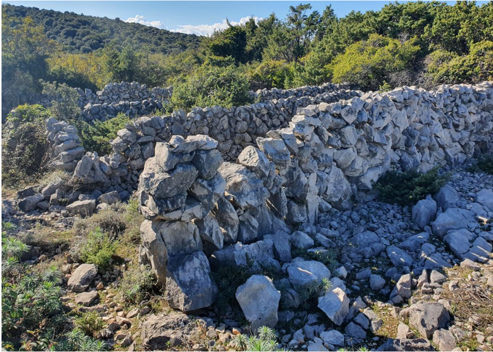
Figure 46. Multicellular sheepfold on Betkav is mostly built of single and combined walls (2020).
