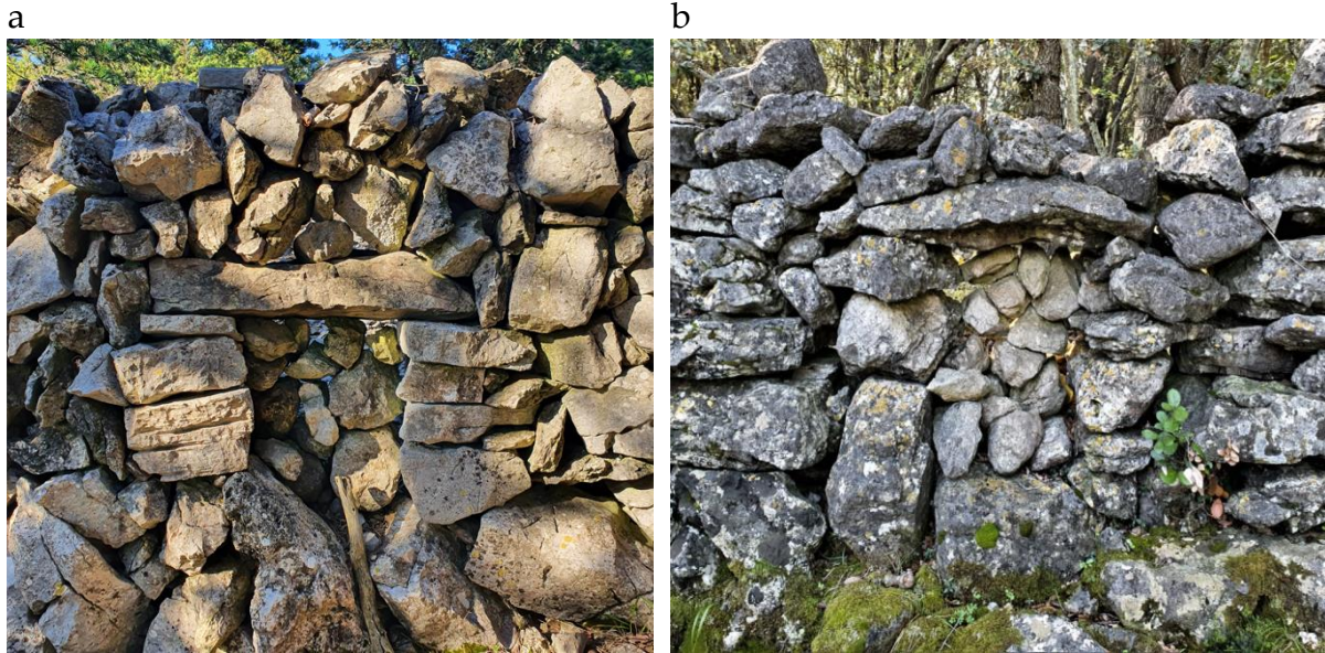
Figure 109. Lunky holes ( škùja ) closed with stones a) on the pathway between Germov and Miholaščica (2021) and b) between Halmac and Veli Tržić (2020)
