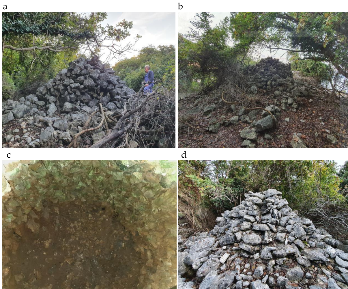
Figure 103. An assumed lime kiln close to Veli Bok (Tramuntana): a) The height of the structure above earth is about 2 m. b) Advanced vegetation and earth mounds prevented the whole dry stone structure from being captured. c) Missing stone from the upper part of the structure enabled the top perspective view, which shows a spacious area within. d) The recognisable 'stone pyramid' shape of the lime kiln can be seen. (2021)
