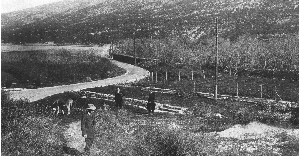
Figure 57. The canals in Piskel in 1910 (Cres Library archive).
