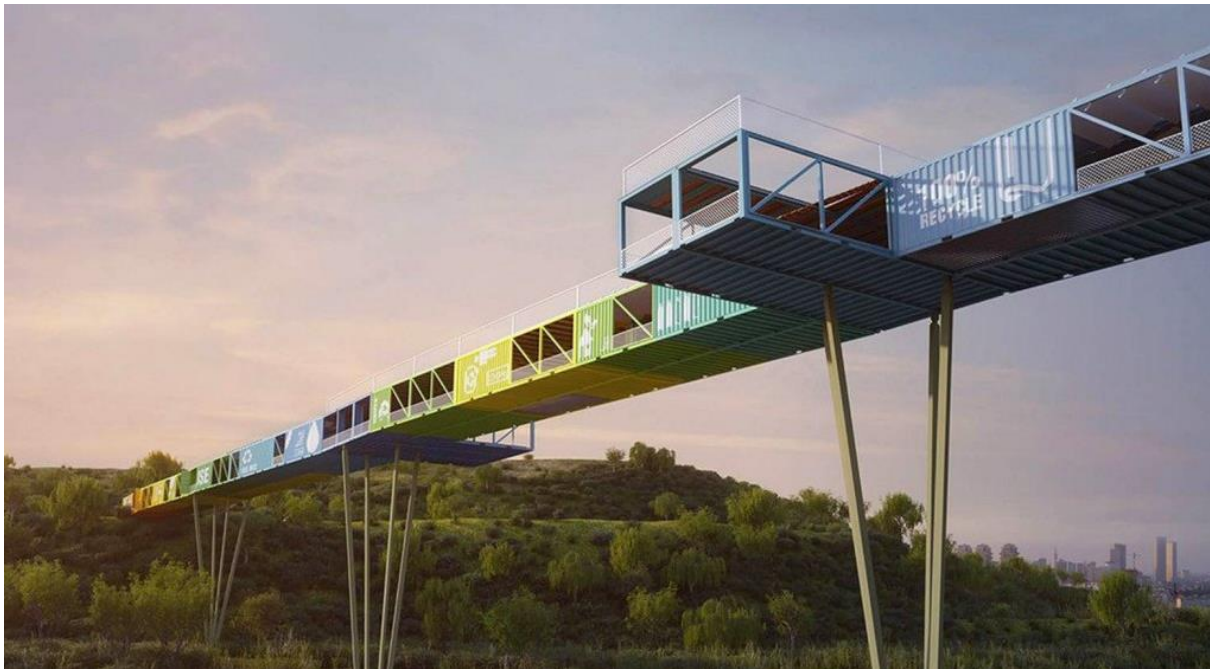
Slika 37: Most od kontejnera ( https://inhabitat.com/econtainer-recycled-shipping-container-bridge-to-provide-gateway-to-tel-aviv-arial-sharon-national-park/ )
