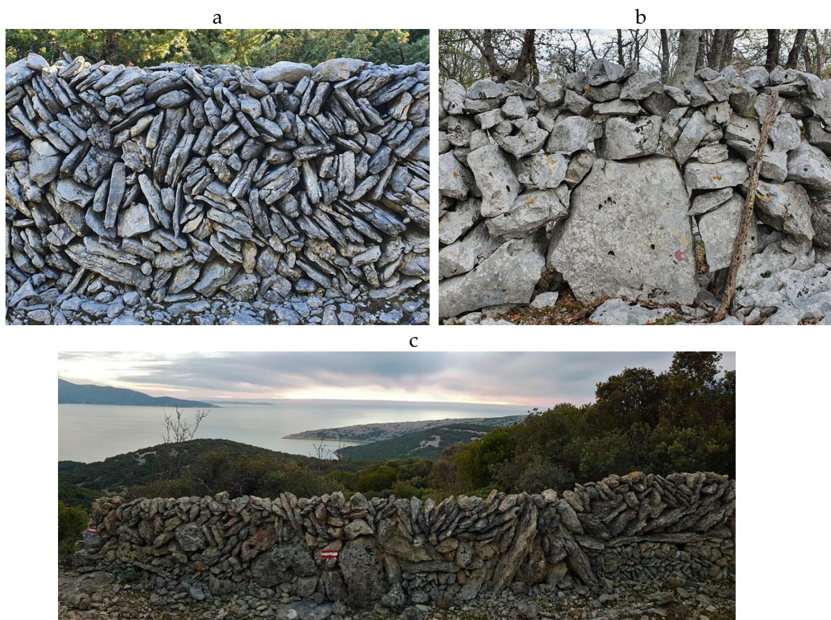
Figure 6. Different forms of dry stone walling reflect dry stone artisans’ craftsmanship, the micro-climate, and the local lithology a) along the pathway between Cres and Loznati (2021), b) on the pathway close to Dragozetići, c) Along the pathway below Ustrine (2019).
