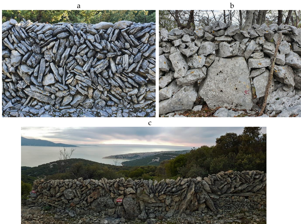
Figure 6. Different forms of dry stone walling reflect dry stone artisans' craftsmanship, the micro-climate, and the local lithology a) along the pathway between Cres and Loznati (2021), b) on the pathway close to Dragozetići, c) Along the pathway below Ustrine (2019).
