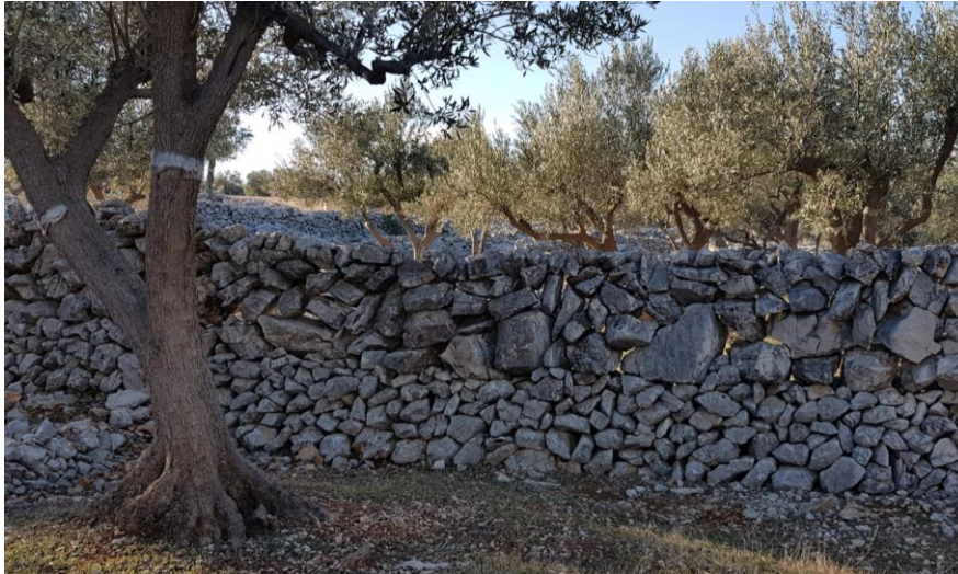
Figure 18. A combined dry stone wall in the town of Cres olive grove, possibly built after the introduction of sheep in 1950s (2019)
