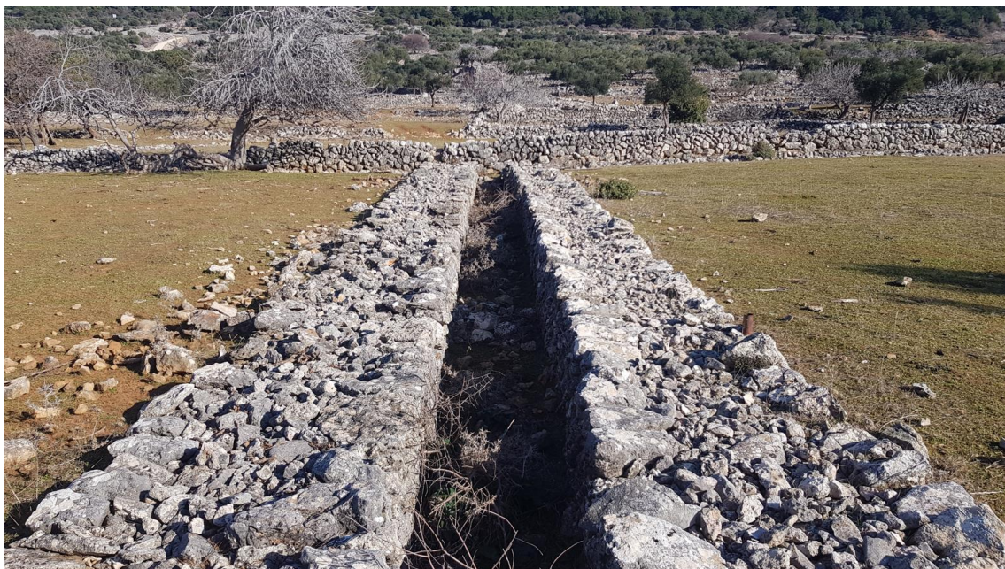
Figure 65. The drainage canal in the fields (Poje, 2019)
