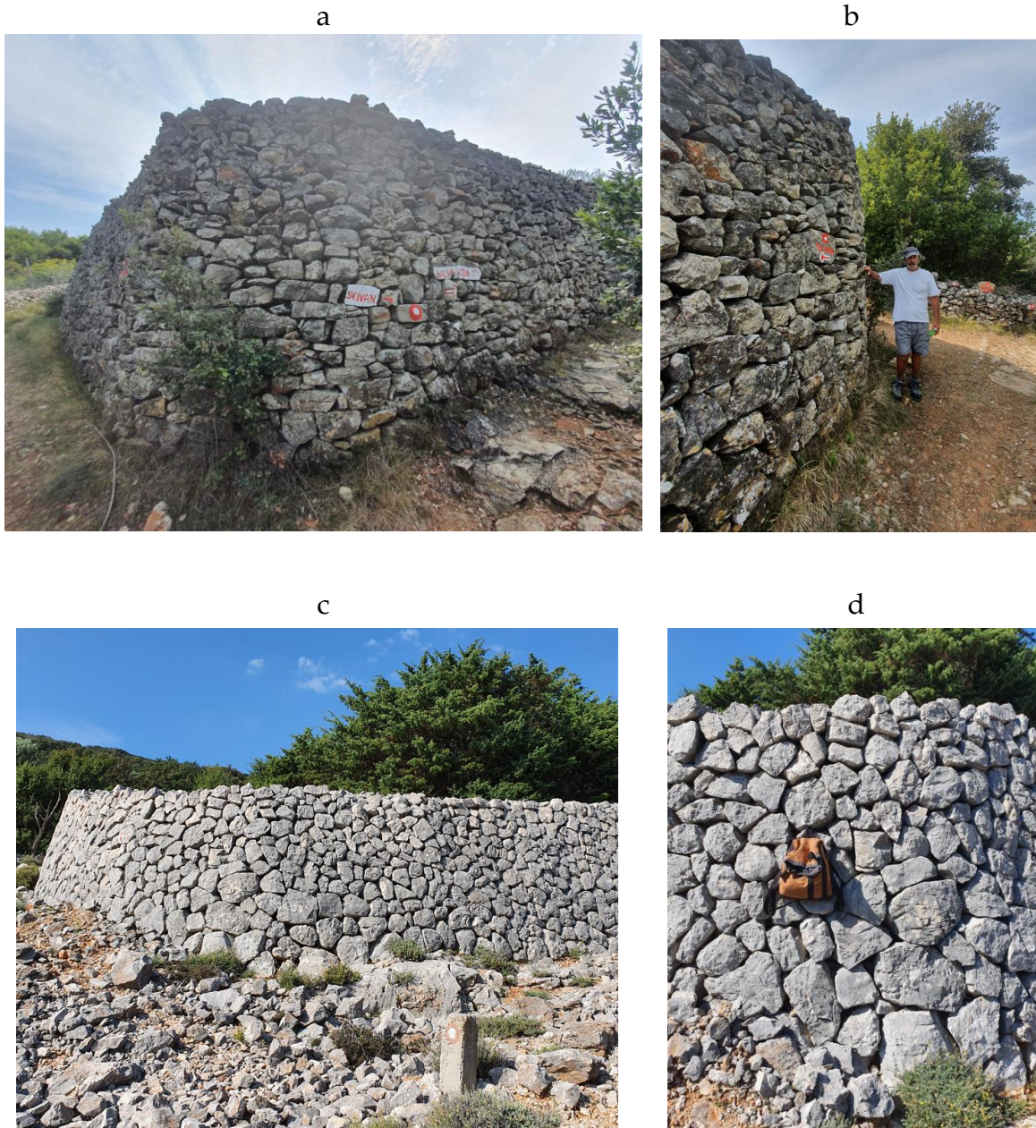
Figure 7. Rare examples of hewn dry stone structures on the Cres and Lošinj islands. These outer walls represent the lower retaining walls a-b) along the pathway from Veli Lošinj to Sveti Ivan (2020) and c-d) Along the gravel road from Cres to Valun (2020)
