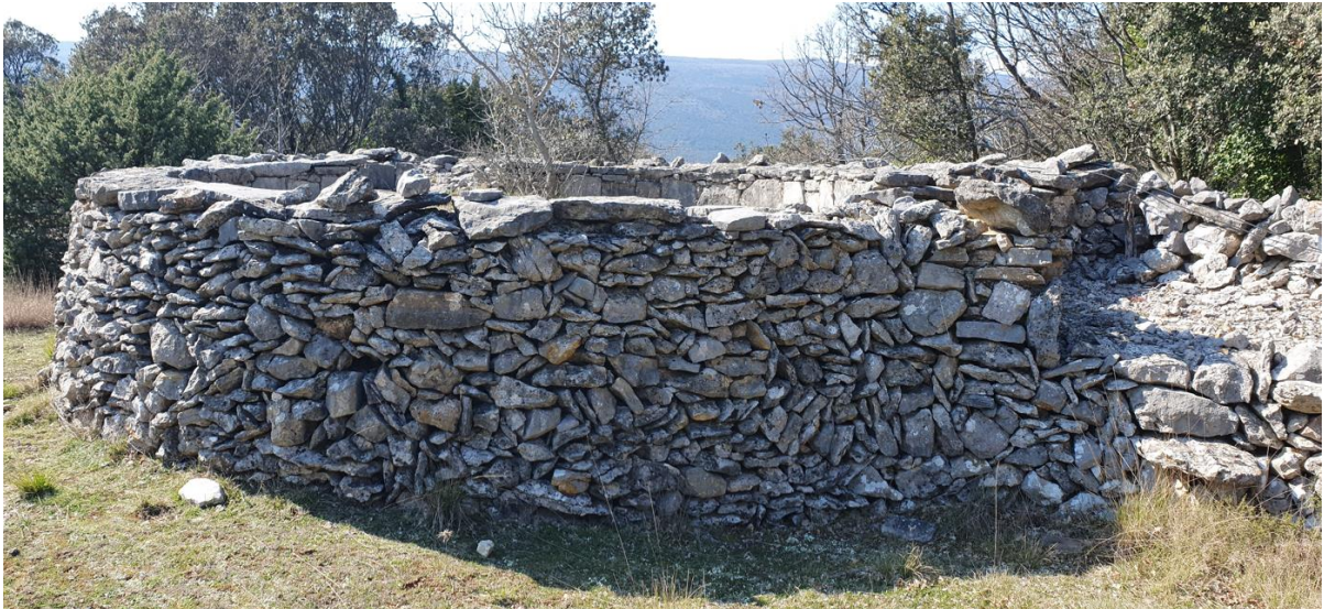
Figure 122. Different perspectives and constructive details of the threshing floor below the village of Stanić (2021)
