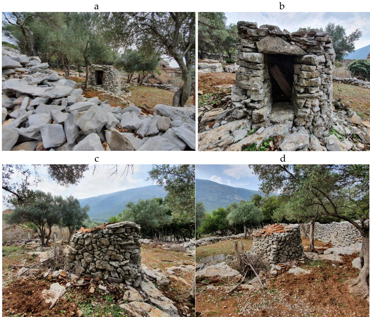
Figure 102. A dry stone water closet, part of one of the buildings in Veli Tržić (a-d), partially covered with stone slabs and roofing tiles (2021)
