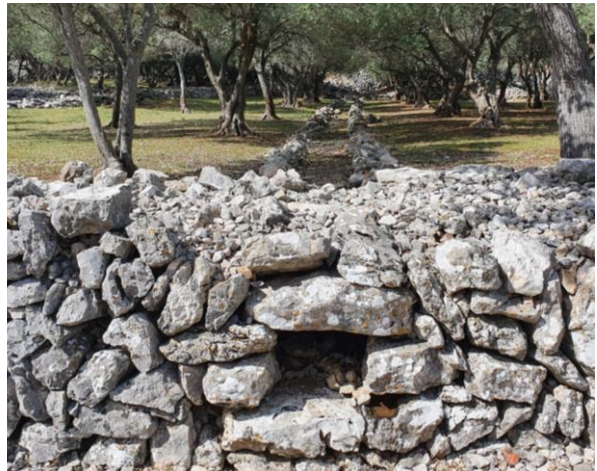
Figure 63. A water conduit funnelling excess water from the agricultural parcels to the street a) near Halmac b) and on Piskel (2020)
