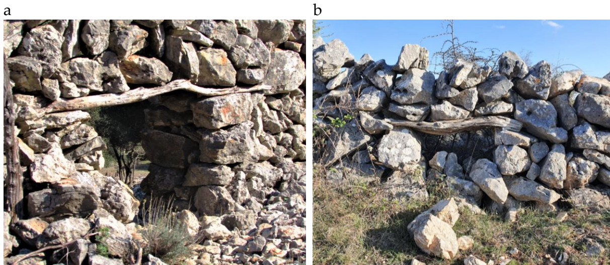
Figure 108. Lunky holes ( škùje ) covered with wooden lintels a) on the ‘Napoleon road’ north of the town of Cres (2017) and b) on the pathway to Zbišina (2021)
