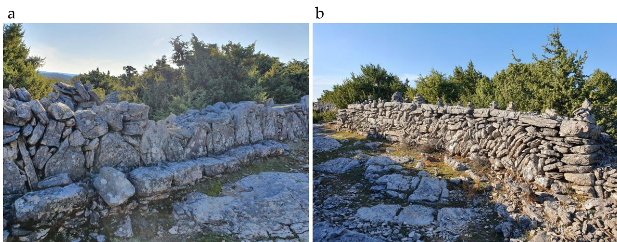
Figure 80. Pocivalić on the path connecting the village of Loznati and Cres: a) The left side of the path had additional steps, probably for the villagers, b) while on the right was pocivalić for the burden. The rocks stacked above are not functional; they were placed by the hikers and tourists afterwards (2021).
