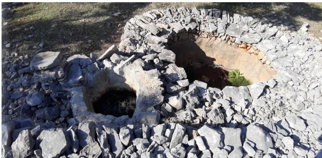
Figure 120. Vaške in the vineyards came in pairs; the larger one was used to collect rainwater, and the smaller one was used for pesticide preparation (© Karla Glavočić, 2019)
