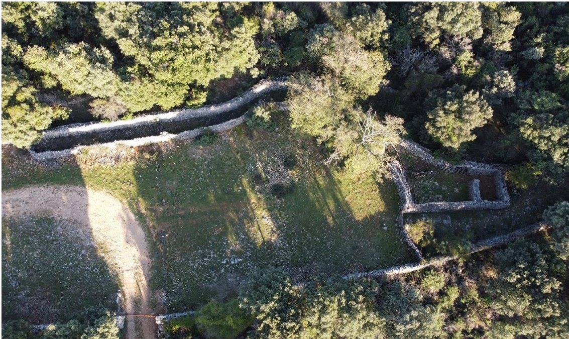
Figure 47. The multicellular sheepfold below the village of Loznati (2021). This sheepfold has an elongated shape, which is relatively common in the southern part of the island of Cres, where long cells are referred to as 'kanūal' (2021)
