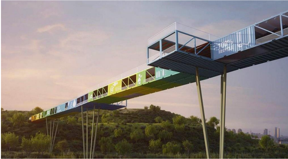
Slika 37: Most od kontejnera ( https://inhabitat.com/econtainer-recycled-shipping-container-bridge-to-provide-gateway-to-tel-aviv-arial-sharon-national-park/ )
